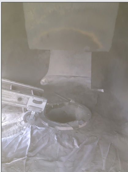
Figure 11. Primary sampling conveyor is pushed through the opening in the dust curtain and placed next to the mouth of the blast hole.
